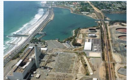
Encina Power Station, Carlsbad
