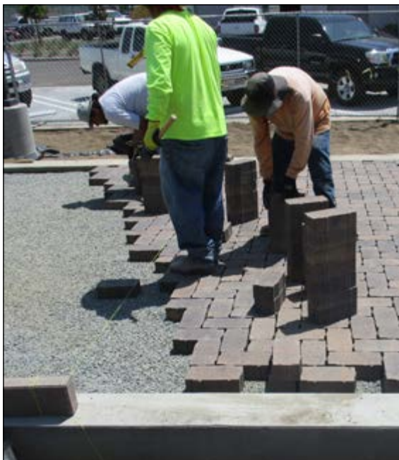
Installation of pervious pavers to reduce runoff to storm drains
