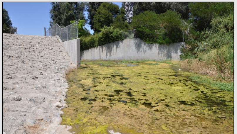
The green alga Cladophora glomerata often proliferates in engineered channels, particularly if nutrient inputs are high and shading has been reduced.
