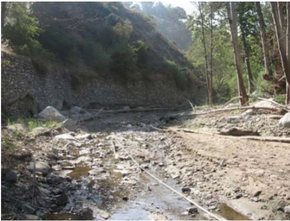
Figure 34. Examples of reaches with one hardened bank. Left: The Arroyo Seco (Los Angeles County). Right: Conejo Creek (Ventura County).
