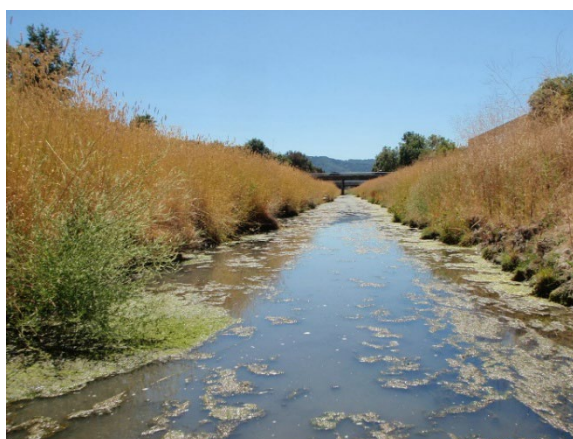
Arroyo Mocho, a soft-bottom modified and straightened channel in Alameda County.
