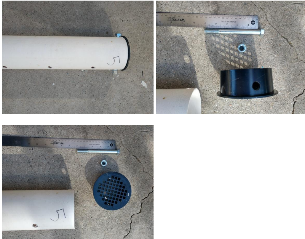
Figure 5.1.1 Example of French drain setup.
