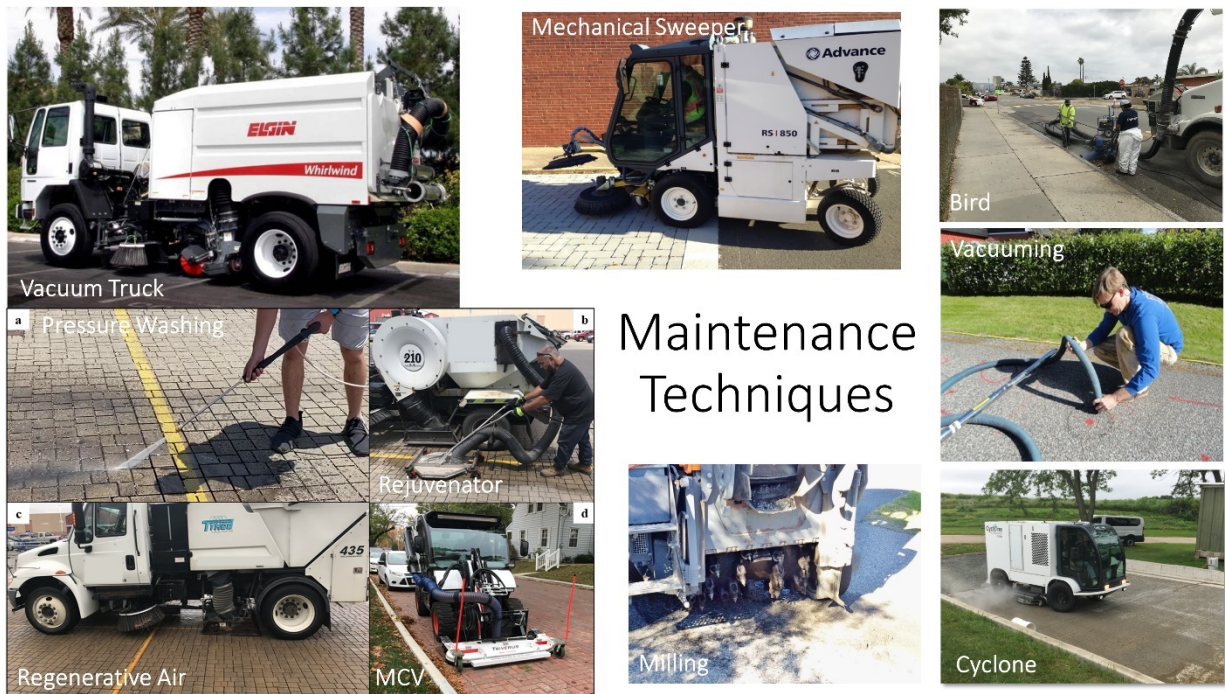
Figure 11. Photographs of routine and restorative maintenance techniques for permeable pavements. Cyclone photograph courtesy Bill Selbig (WI USGS). BIRD photograph courtesy: Count of Ventura Public Works.
