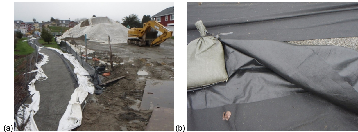
Figure 6. Pervious concrete sidewalks in Seattle in 2008; (a) at high risk of clogging due to adjacent sediment stockpile and poor erosion and sediment controls; (b) attempts to protect pervious concrete during construction by wrapping in HDPE and geotextile secured with sand bags.
