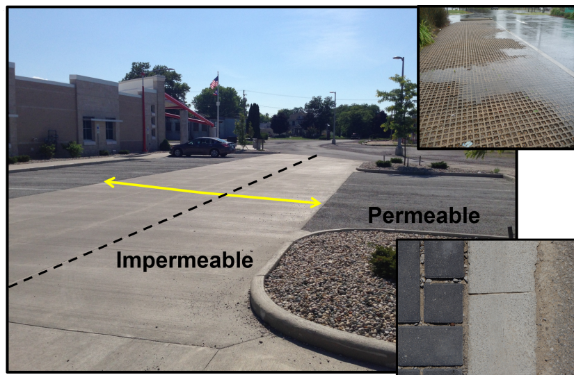
Figure 3. The permeable / impermeable interface (PII) with several photos of clogging at these locations.
