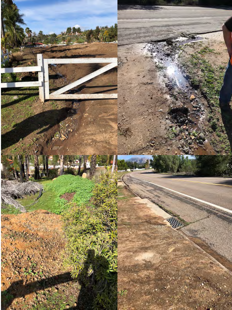
Figure 2. Clockwise from top left: Horse corral with disturbed leach field and drainage ditch; Discharge from drainage ditch to street; piles of manure adjacent to street; catch basin in street between the drainage ditch discharge and the manure piles.
