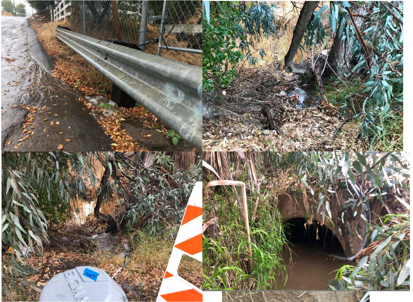
Figure 1. Clockwise from top left: Curb runoff upstream of the LC8K outfall; LC8K outfall to Flinn Springs Creek ; LC8K outfall with storm water flowing; LC8K outfall dry showing sediment inundation and sampling tubing; Sample collection site with pump and tubing leading to LC8K outfall and pump setup at LC8K outfall.
