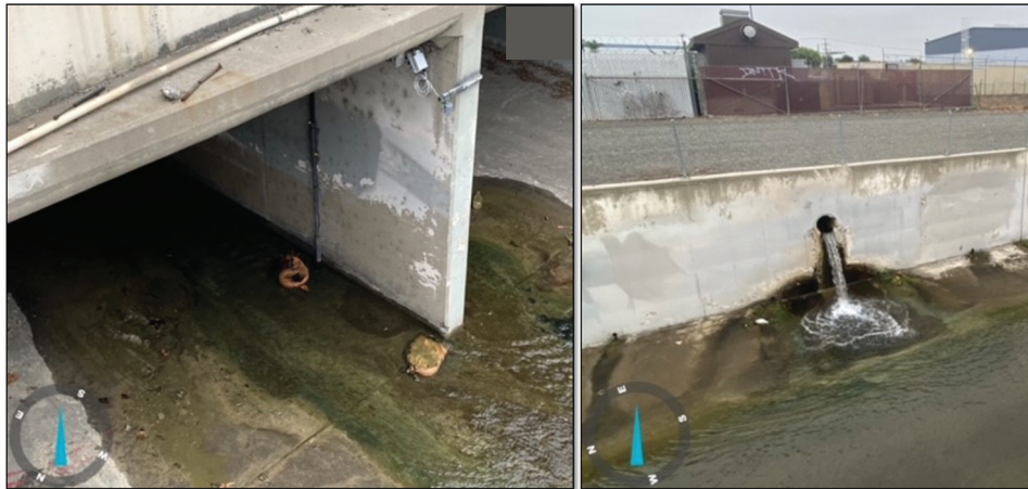
Figure 8. Evidence of a discharge during the all-Hands Week follow-up visit at Site C for alarm on October 16, 2024. The elevated discharge at the monitoring station (left) was traced to an outfall upstream (right). Photos used with permission from Craig Foster, City of Santa Ana.
