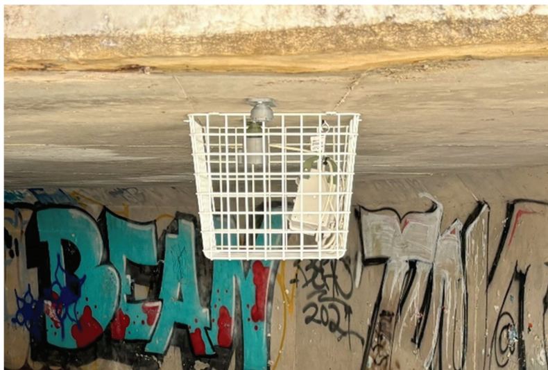
Figure 4. Cages were deployed at some sites to deter vandalism/theft of RAD and CAM sensors.
