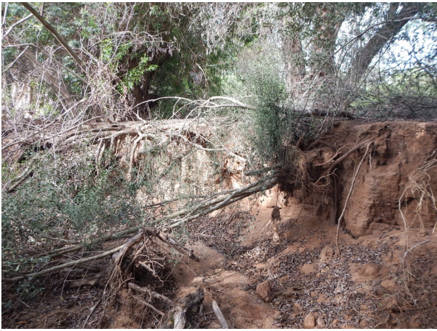
Fig. 7 Typical southern California example of incision and bank failure observed in fine-grained channels downstream of conventional development (27% TIA, developed in the 1980's) that lack stormwater intervention tailored at reducing sediment transport capacity
