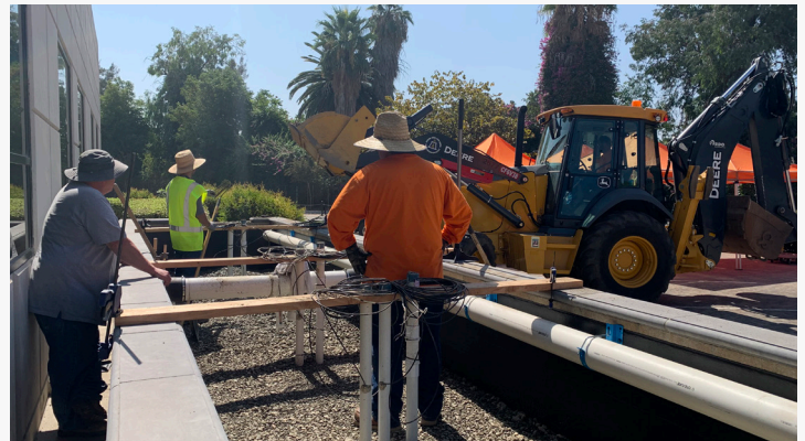
A biofiltration BMP under construction in Riverside County
