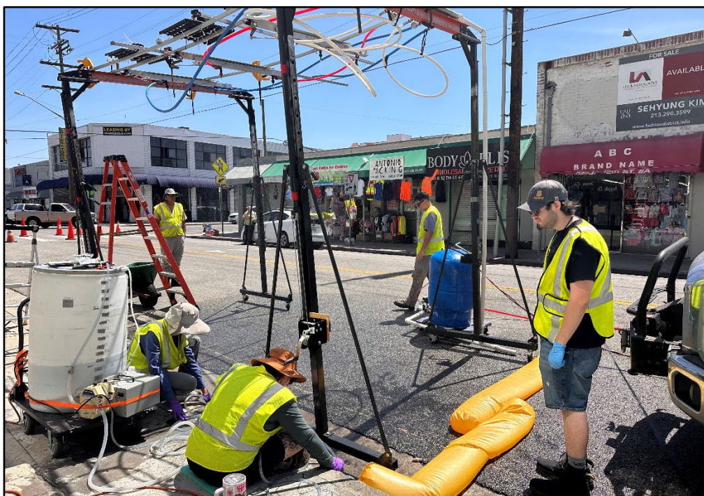
A SCCWRP field crew sets up a custom-built rainfall generator on a commercial street in Los Angeles, part of an ongoing study to measure the efficiency of routine street sweeping in removing pollutants that would otherwise enter storm drains and contribute to runoff pollution.
