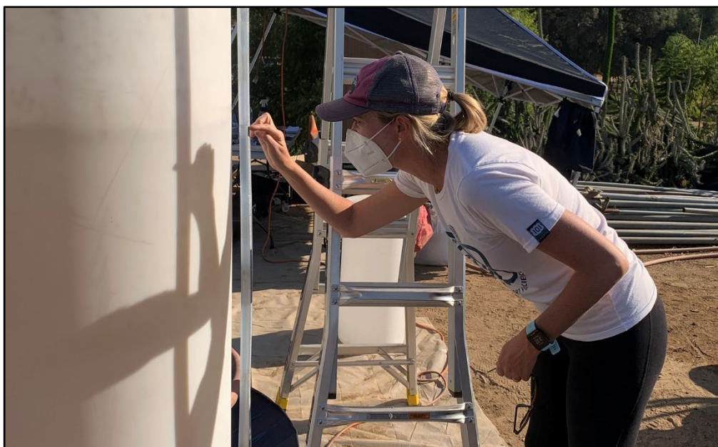
A field crew inspects a stilling well that is being used to measure how much water was recovered after being pumped through a segment of sewer pipe in San Diego. The novel exfiltration measurement method was piloted during a recent SCCWRP-led study that quantified sources of fecal contamination in the urbanized lower San Diego River watershed during wet weather.
