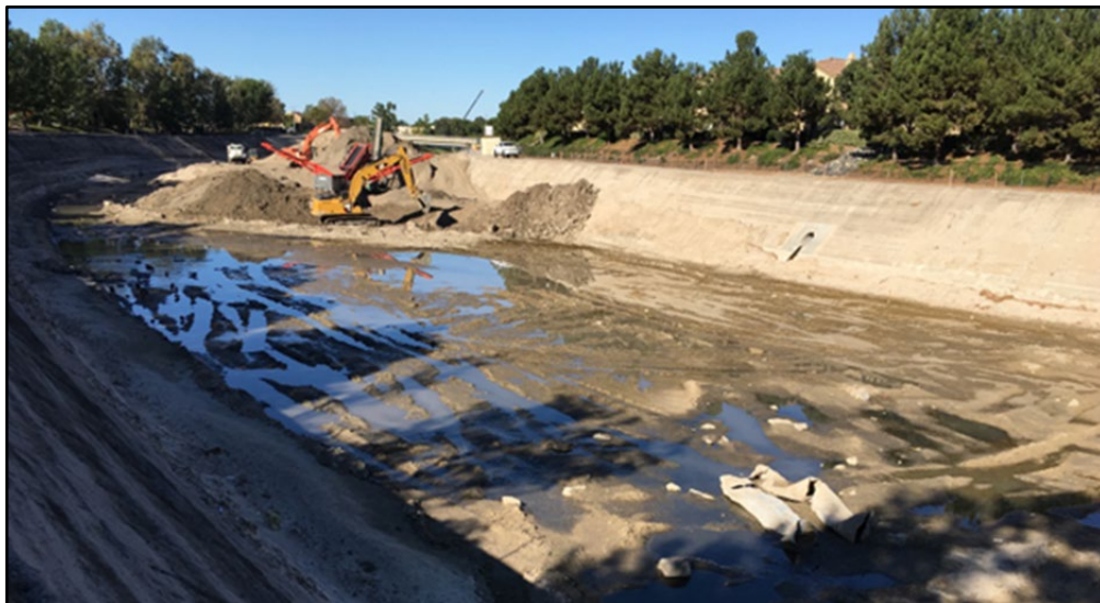
SCCWRP and the Southern California Stormwater Monitoring Coalition have begun working to understand how to protect and restore the biological health of Southern California's engineered channels, including this one, above, that depicts a field crew removing accumulated sediment as part of channel maintenance. The study will examine whether physical habitat restoration strategies can be expected to improve stream biological health.
