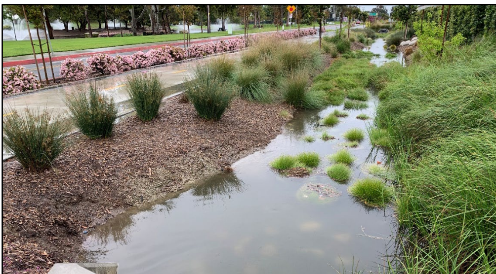
A bioswale that runs along the side of a roadway in Orange County collects and treats stormwater runoff. SCCWRP has developed a scoring tool known as the Multi-Metric BMP Performance Index to quantify the performance of structural BMPs and provide insights into whether they are performing at levels that contribute to meeting watershed-specific water-quality goals.
