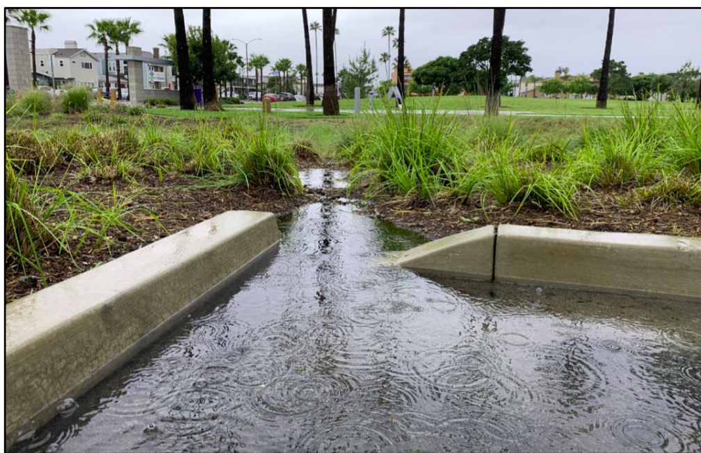
Runoff from a parking lot drains to a bioretention system containing special engineered soil media designed to remove contaminants. A SCCWRP-hosted international conference scheduled for January 2022 will provide a forum for advancing modeling of urban stormwater drainage systems.
