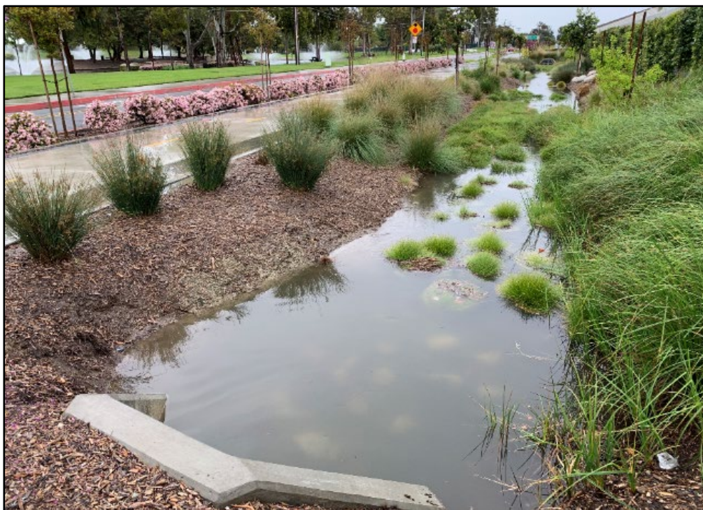
A bioswale that runs along the side of a roadway in Orange County collects and treats stormwater runoff. The Southern California Stormwater Monitoring Coalition (SMC) has begun building a regional monitoring network to track the performance of a wide variety of bioswales and other stormwater BMPs.
