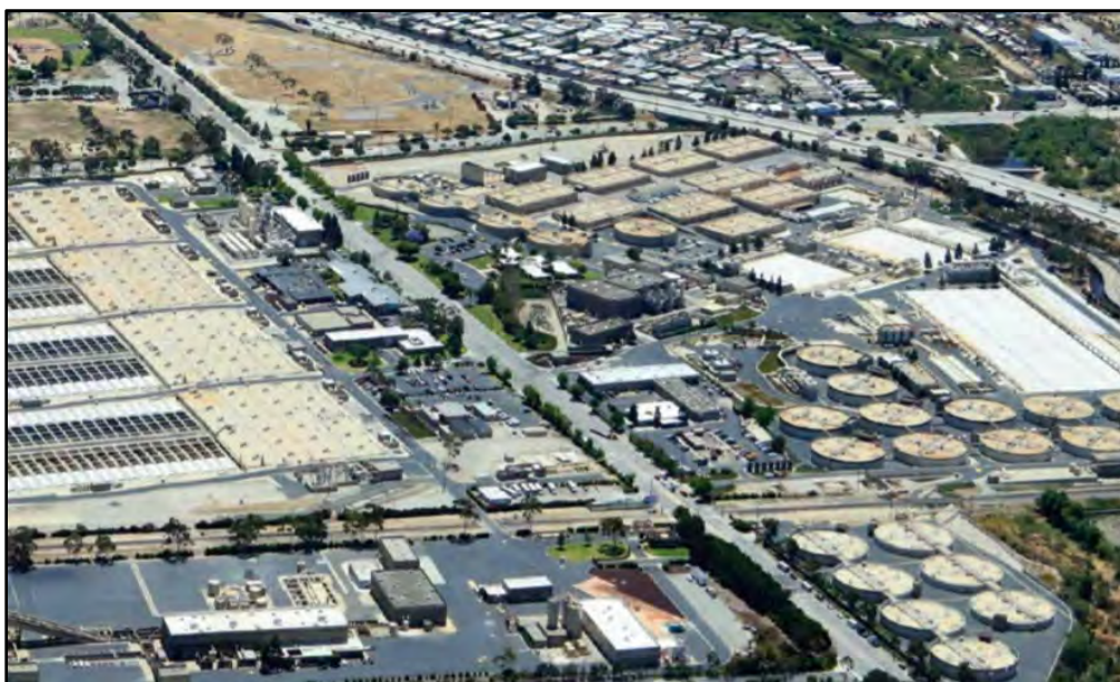
Photo courtesy of Sanitation Districts of Los Angeles County
