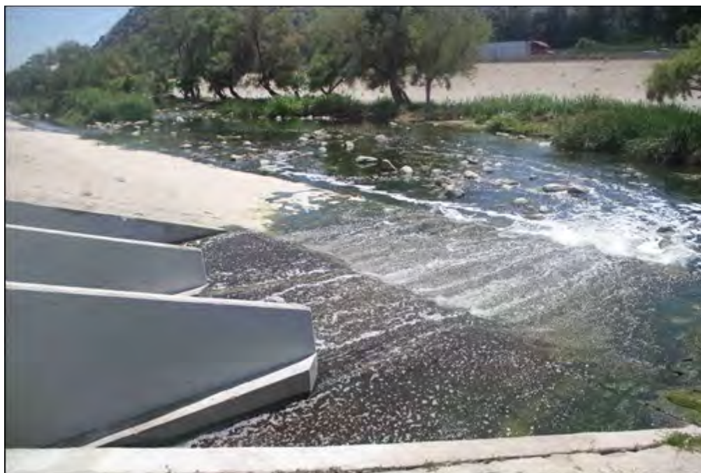
Treated wastewater effluent is discharged into the Los Angeles River from the nearby L.A.-Glendale Water Reclamation Plant. Water-quality managers for the effluent-dominated river are exploring the potential ecological and recreational effects of diverting effluent and runoff from the river for water recycling purposes.
