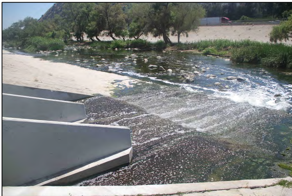
Treated wastewater effluent is discharged into the Los Angeles River from the nearby L.A.-Glendale Water Reclamation Plant. Water-quality managers for the effluent-dominated river have initiated a study to explore the potential ecological and recreational effects of diverting effluent and runoff from the river for water recycling purposes.
