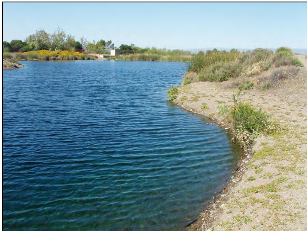
Recycled water is sometimes placed into holding ponds, such as this one in Santa Clara County in Northern California, to allow the water to gradually infiltrate into groundwater. California's policy on how to monitor CECs in recycled water was recently revisited by an expert advisory panel facilitated by SCCWRP.
