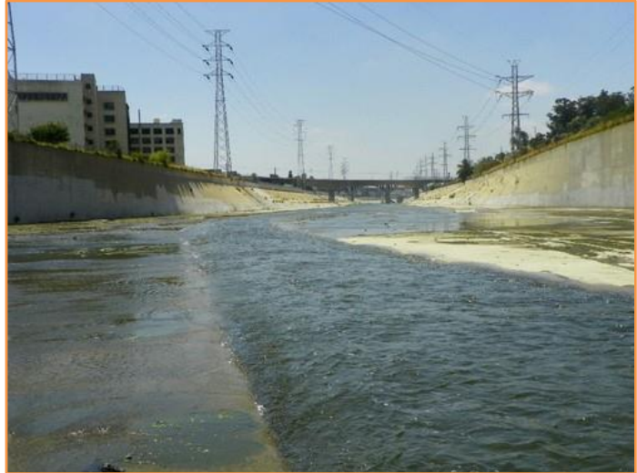
Treated effluent is released into the highly channelized Los Angeles River. SCCWRP has designed a study that will monitor for CECs in this type of environment.
