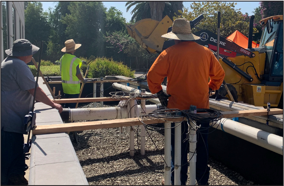
A field crew constructs a bioretention planter in Riverside County to study its mechanistic inner workings. California is evaluating the potential for stormwater BMPs – specifically, bioretention and biofiltration systems – to filter and remove microplastics and other pollutants from runoff.
