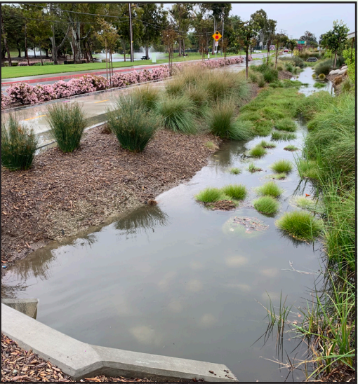
A bioswale that runs along the side of a roadway in Orange County collects and treats stormwater runoff. SCCWRP and its partners have launched a study to characterize the mechanistic inner processes by which biofiltration BMPs remove common contaminants in runoff.
