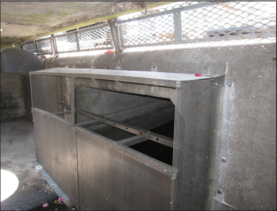
Courtesy of Los Angeles County Department of Public Works Metal mesh screens help block trash and other debris from entering storm drain pipes just below street level. These trash-capture devices are a key part of Southern California’s next-generation strategy to combat trash pollution.
