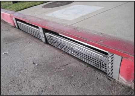
Courtesy of Los Angeles County Department of Public Works Metal mesh screens have been installed at thousands of storm drain inlets across Southern California over the past decade to combat the introduction of trash into aquatic environments. The screens, above, open automatically when obstructed by debris to prevent flooding.
