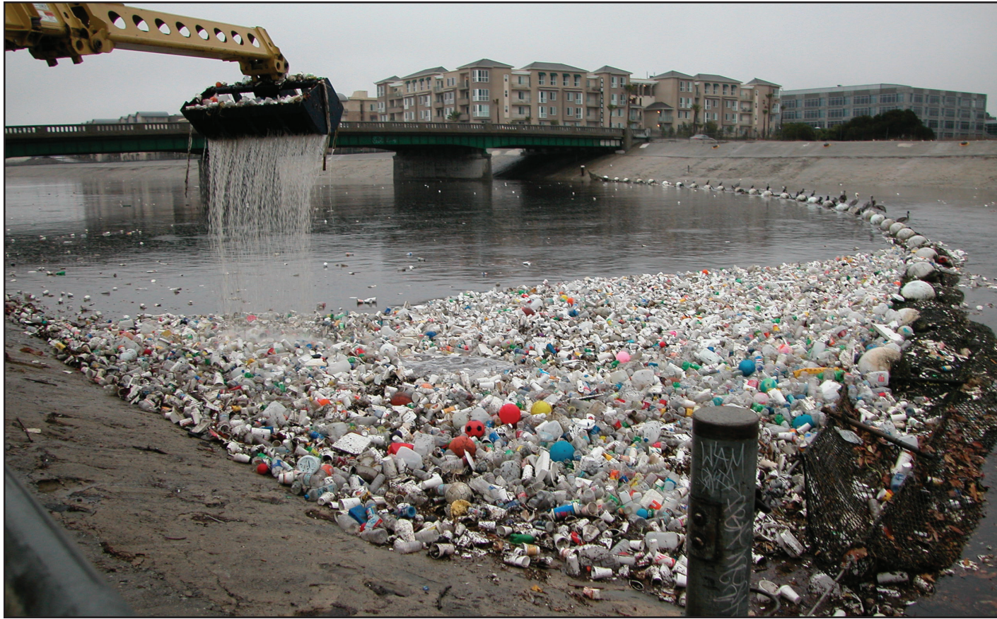
Trash booms at the mouth of Ballona Creek in Los Angeles capture floating debris before it reaches the coastal zone. An analysis by the Bight and SMC regional monitoring programs found that total trash levels in Ballona Creek and the other waterways draining to Santa Monica Bay dropped nearly tenfold following full implementation of a regulatory program to combat trash loading.
