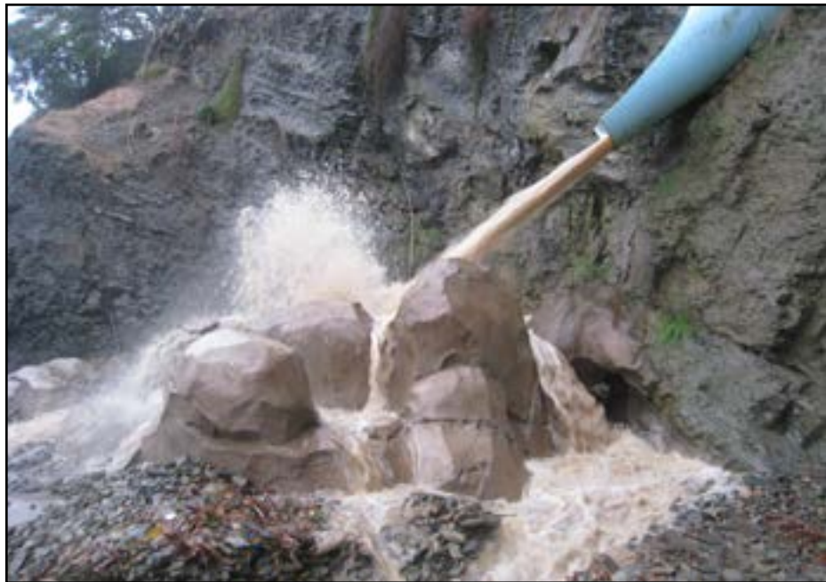
Stormwater pours out of a drain that terminates at the coastal zone. Southern California’s storm drain system transports litter to coastal waters from across hundreds of square miles.
