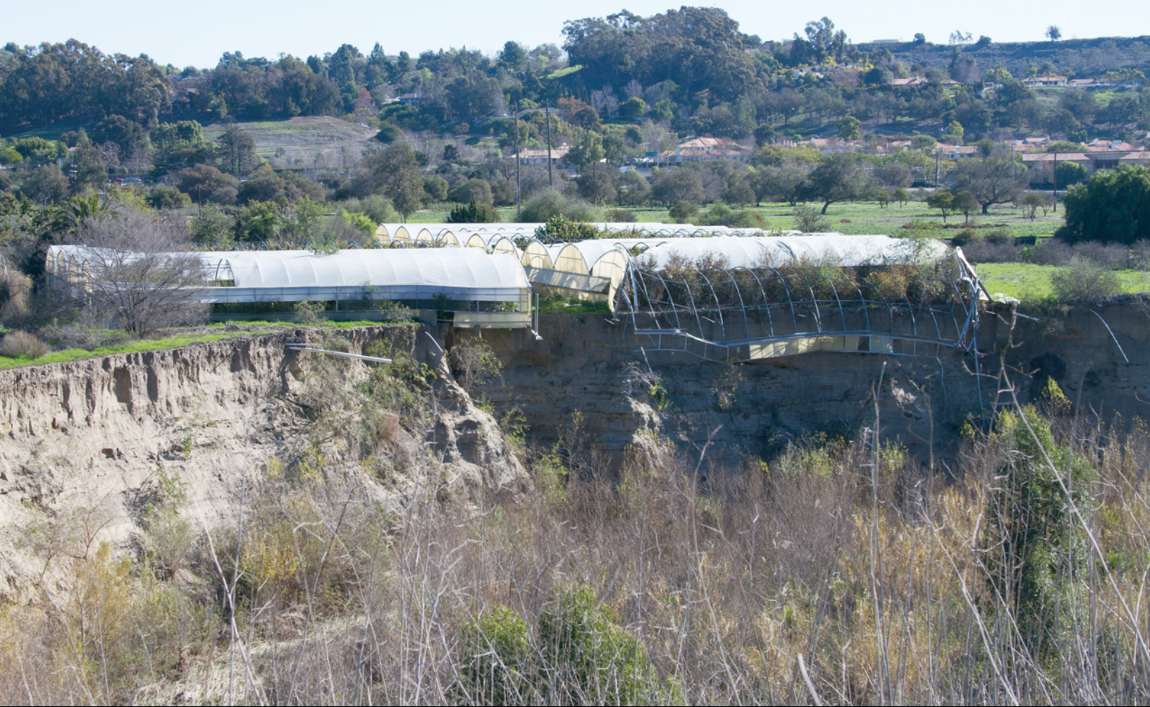
A nursery greenhouse perches precariously atop an eroded bluff in Oso Creek in southern Orange County. Although water levels in the creek do not reach the greenhouse itself, the base of the creek walls have been eroded, causing the earth above to give way.
