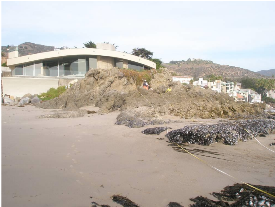
Figure B-8. Lechuza Point is comprised of bedrock and sand with moderate relief. The surrounding coast is made up of bedrock and sand. The survey area is divided into two sections. The upcoast section is 14 meters wide and 45 meters long. The biological community at this site differs from that expected based on other sites in the region. It is likely that this is due to the influence of sand burial and scour at the site.
