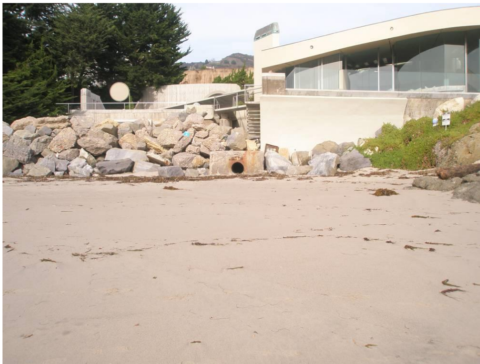
Figure B-10. The nearest storm water discharge pipe to Lechuza Point is 25 meters from survey bolt OT1.
