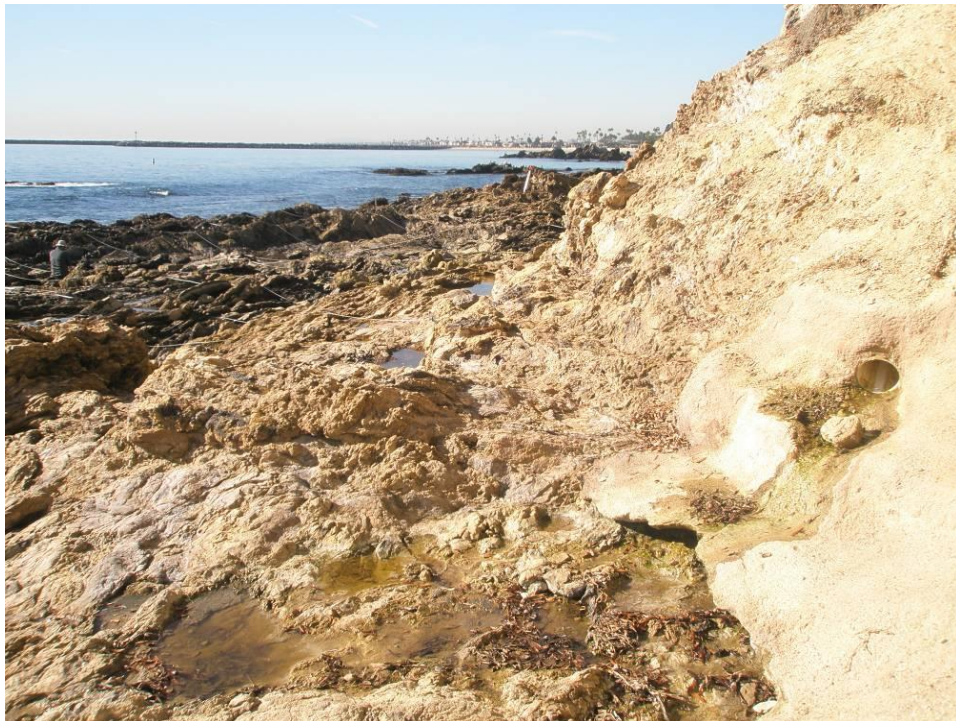
Figure B-16. The nearest storm water discharge pipe (NEW016) to Buck Gully South is 5 meters from survey bolt OT2.
