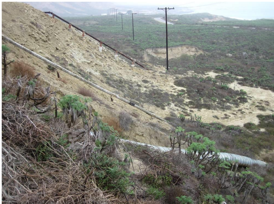
Figure B-31. The nearest storm water discharge to Tranquility Beach is approximately 100 meters from survey bolt OT1.
