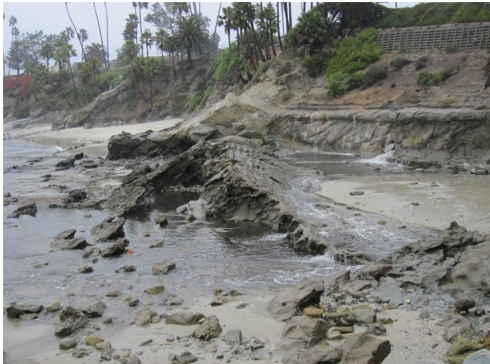
Figure B-21. The nearest storm water discharge pipe (HSL013) to Heisler Park is 52 meters from survey bolt OT1.
