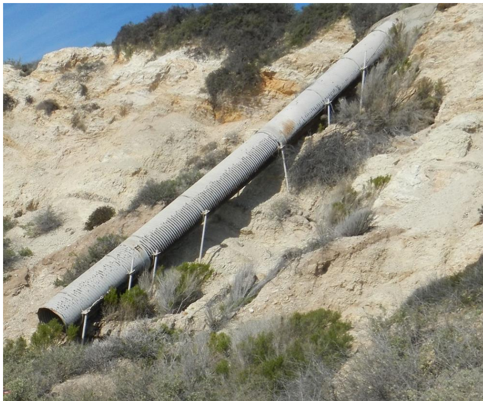
Figure B-19. The nearest outfall (IRV009) to Muddy Canyon is approximately 207 meters downcoast of the survey bolt OT2.
