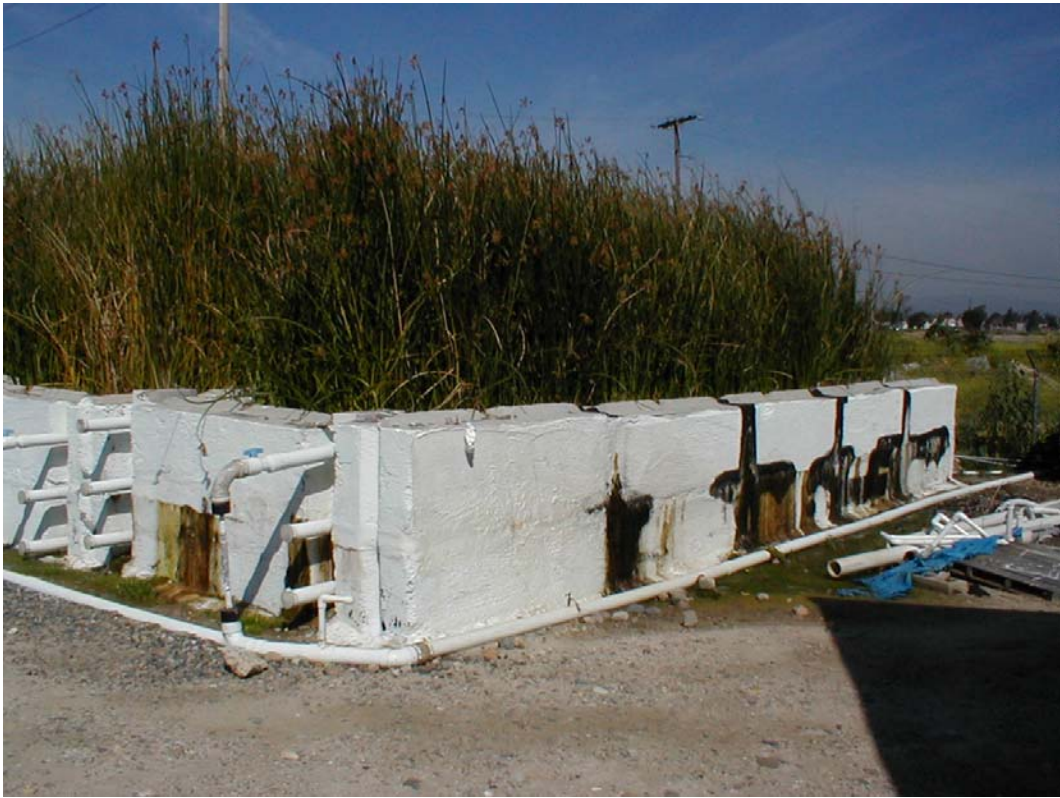
Figure 3. Orange County Water District's sub-surface flow wetlands. These wetlands are constructed from concrete panels, and measure approximately 1 m tall x 2 m wide x 8 m long. Each wetland cell is filled with a gravel matrix composed of pea gravel. A monoculture of wetland plants (bulrushes, genus Scirpus ) are planted in the gravel. The gravel provides an approximate thousand-fold increase in surface area for the growth of bacterial biofilms that increase the rate of contaminant degradation or removal. Within the gravel matrix there are distinct oxygen rich (aerobic) and oxygen free (anaerobic) zones where specific microbial processes take place. Water flows beneath the surface of the gravel matrix.
