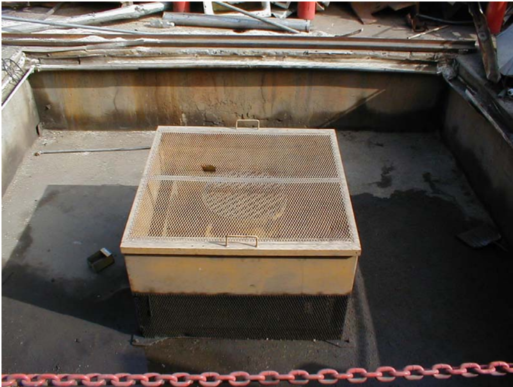
Figure 10. L.A. metal recycling yard BMP. Water flows through the grating of the metal top hat, into an infiltration trench.
