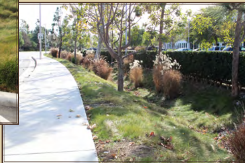
Vegetated swales allow parking lot runoff to infiltrate on-site.
