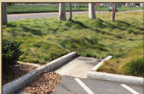
Vegetated swales allow parking lot runoff to infiltrate on-site.
