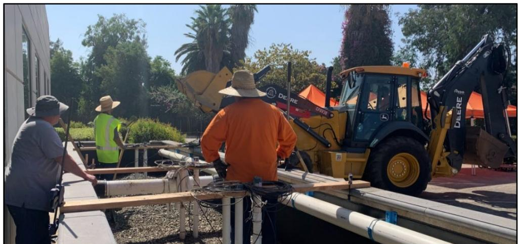
**A field crew constructs a bioretention planter in Riverside County to study its mechanistic inner workings. The Southern California Stormwater Monitoring Coalition (SMC) has collected performance data of structural stormwater BMPs (best management practices), like bioretention planters, at five sites – a key milestone in ongoing efforts to build the SMC's new Regional BMP Monitoring Network.**
