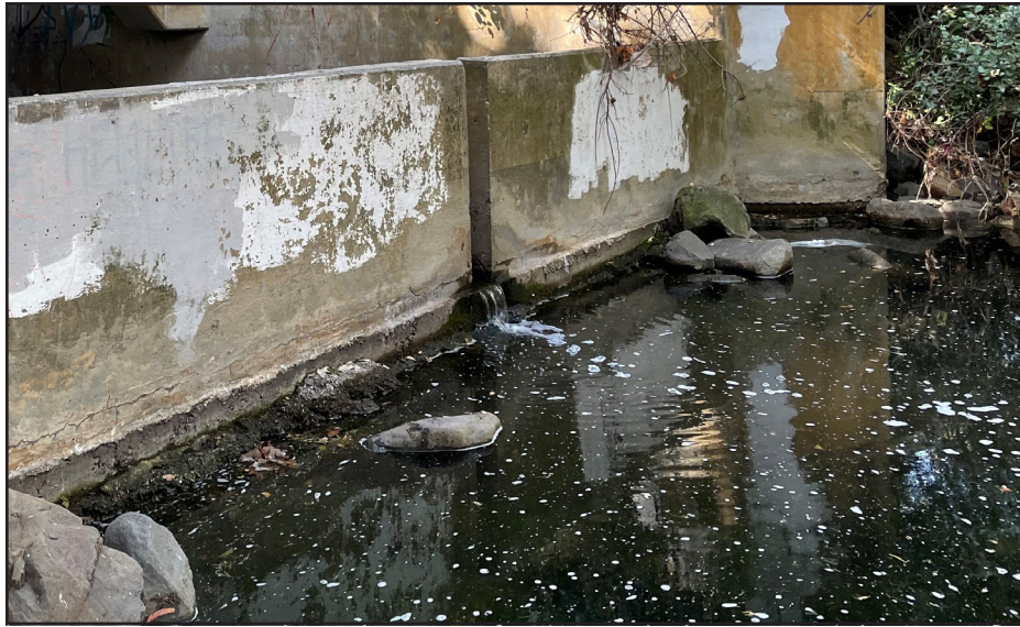
A storm drain discharges unnatural dry-weather flows into a tributary of Arroyo Trabuco Creek in southern Orange County. Researchers have used the California Environmental Flows Framework to help local watershed managers decide how they should reverse these unnatural flow patterns, which have degraded stream habitat.
