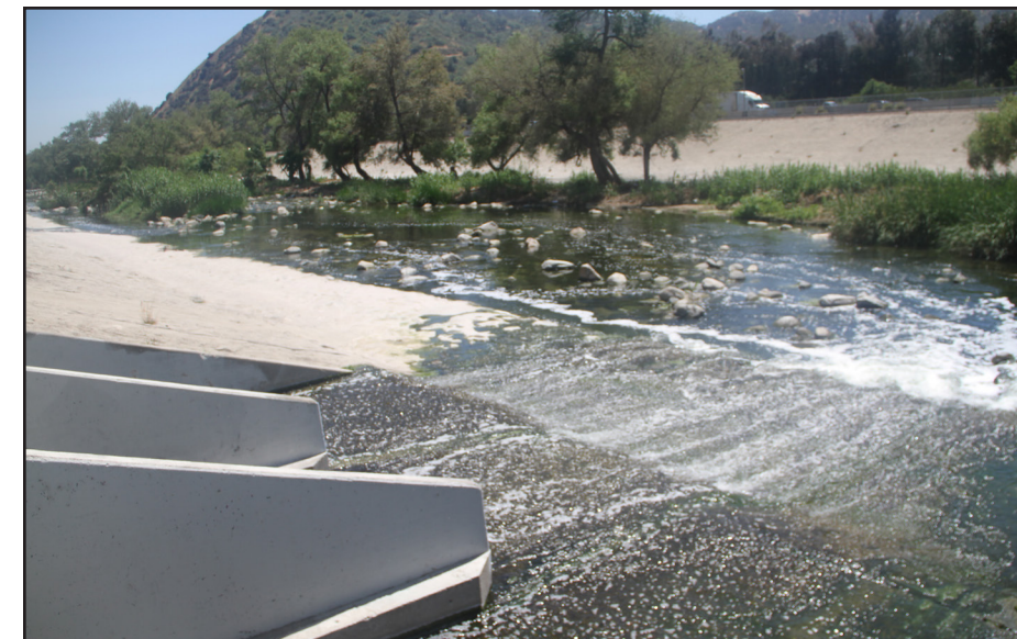
Treated wastewater effluent is discharged into the Los Angeles River from a nearby water reclamation plant. Researchers have developed a standardized approach to help L.A. River managers determine if some of the river's flows can be diverted for water-recycling purposes without jeopardizing the ecological and recreational benefits that these flows provide.
