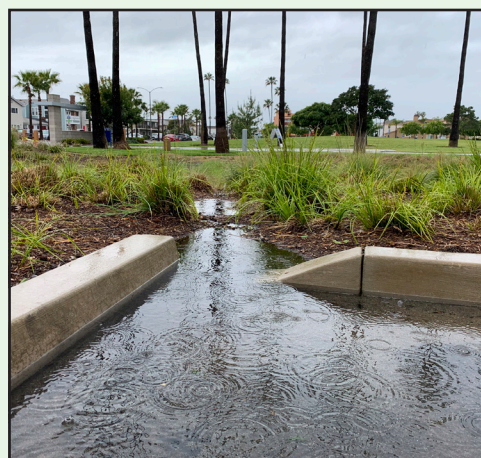
Runoff from a parking lot drains to a bioretention system containing special engineered soil media designed to remove contaminants. Runoff management solutions like this one are the focus of newly developed statewide guidance for how to periodically evaluate long-term, multi-phased plans for improving runoff water quality.
