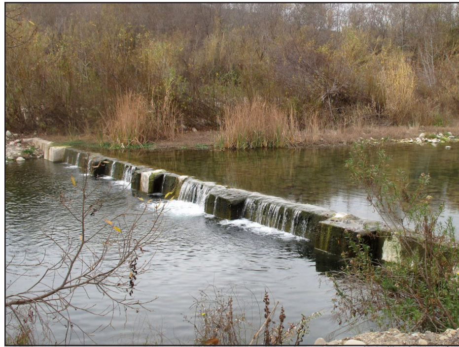
Courtesy of Ventura River Watershed Council Californians have made numerous alterations to the way water flows across landscapes. Above, the Foster Park Subsurface Dam and Diversion in Ventura County is designed to slow the flow of water in Coyote Creek, enabling water to be extracted more readily and improving the efficiency of groundwater recharge.
