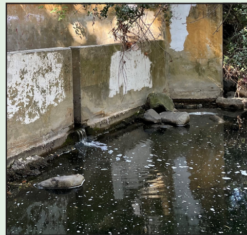
A storm drain discharges unnatural dry-weather flows into a tributary of Arroyo Trabuco Creek in southern Orange County. Researchers have completed a study that sheds light on how stream managers can take a science-informed approach to deciding how they should reverse the area's unnatural flow patterns and improve 23,000 linear feet of degraded stream habitat.
