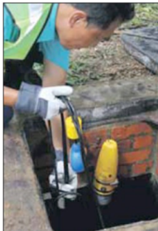
The PUB installed 40 sensors in industrial sites to monitor concentration levels of chemicals discharged into the sewerage system.
